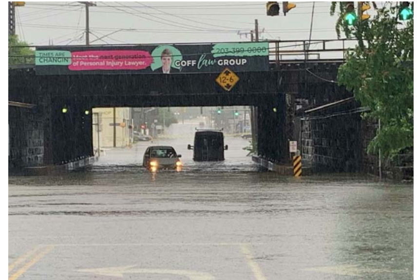
Stamford Advocate https://www.stamfordadvocate.com/local/article/Tropical-Storm-Elsa-causes-heavy-flooding-16303636.php#photo-21217276
